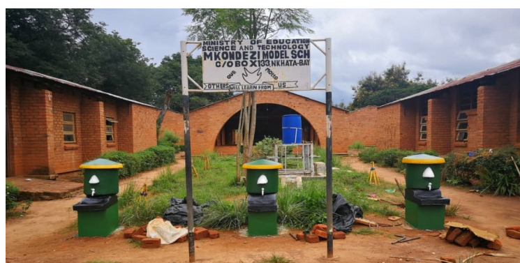
Picture 11: Three out of 80 hand-washing stations. The grey water will be directed towards green areas of the school, to be used for watering.
